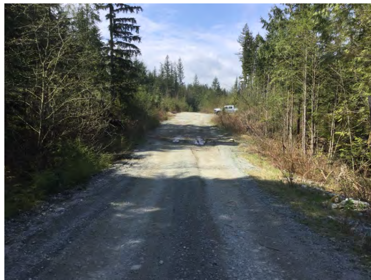
Approach from Right Bank when facing downstream
